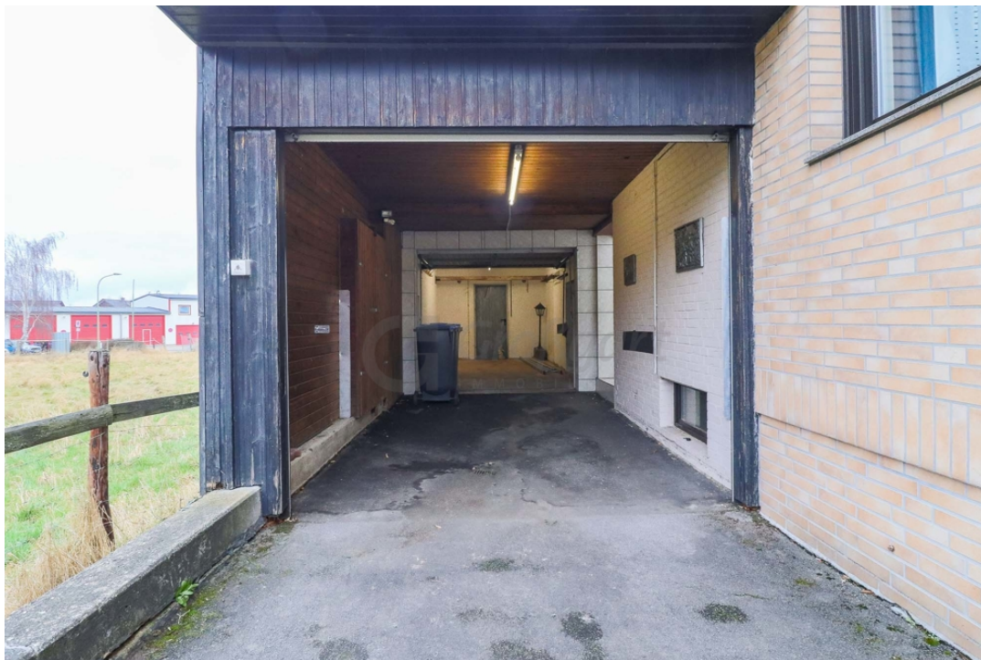
Blick zur Garage
